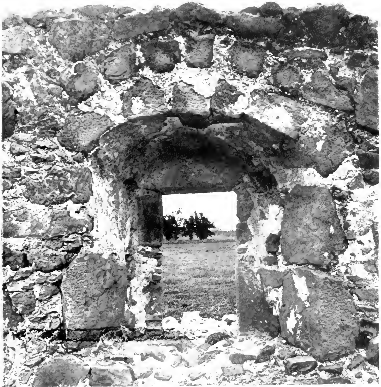
STONE ARCHED DOORWAY, SANTA MARGARITA CHAPEL.
